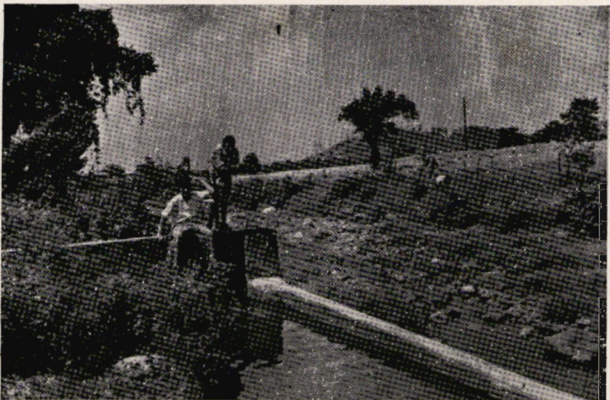
Dam, Río Guamani, Guayama. Sluice gate by means of which water is diverted to Colonia Vives.
